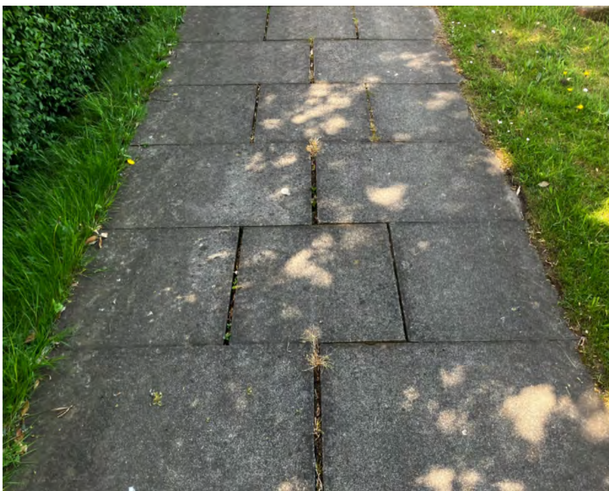
Replace paving slabs to reduce ongoing maintenance liability and trip hazards.
